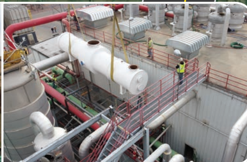
Jackson, NE - Oct. 4th - Fall 2022 Shutdown Replacing the 190 Condenser during our 2022 Fall Shutdown. This vacuum condenser converts vapors into 190 proof liquid ethanol. Weighing in at 86,650 pounds empty! One heavy load!
