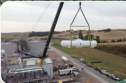
Jackson, NE - Oct. 4th - Fall 2022 Shutdown Replacing the 190 Condenser during our 2022 Fall Shutdown. This vacuum condenser converts vapors into 190 proof liquid ethanol. Weighing in at 86,650 pounds empty! One heavy load!
